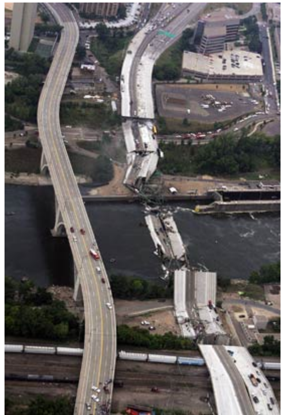
Figure 4. Aerial view of the collapsed bridge in Minneapolis (2 nd August 2007).
