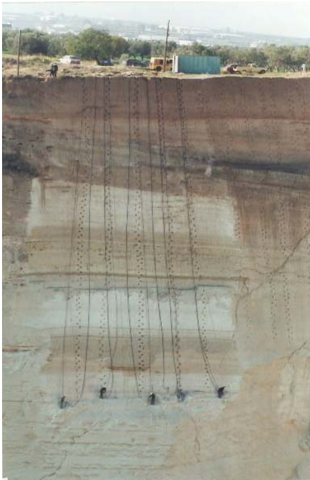
Figure 29. Rehabilitation works on the slopes of the Corinth Canal
