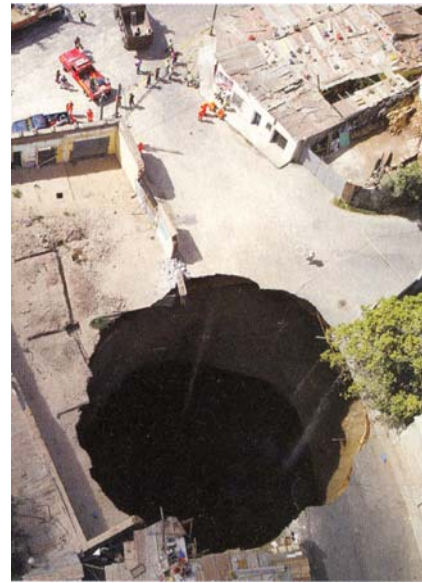
Figure 3. Leakage of a sewer pipe created a hole of 30.5 m diameter and 49 m depth in Guatemala City.
