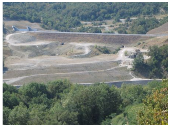
Figure 18. The Anthochori Embankment on the Landslide Area after the Construction of the Remedial Measures.
