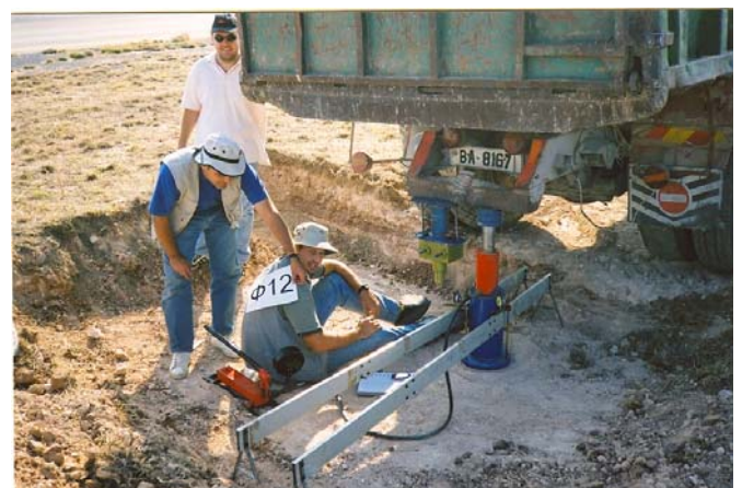
Figure 27. Geotechnical investigations for the rehabilitation of Tanagra airport runway pavement.
