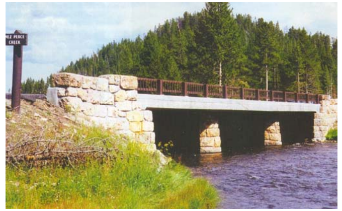
Figure 22. Nez Perce Creek Bridge at the Yellowstone National Park, USA (Barrows et al., 2005).
