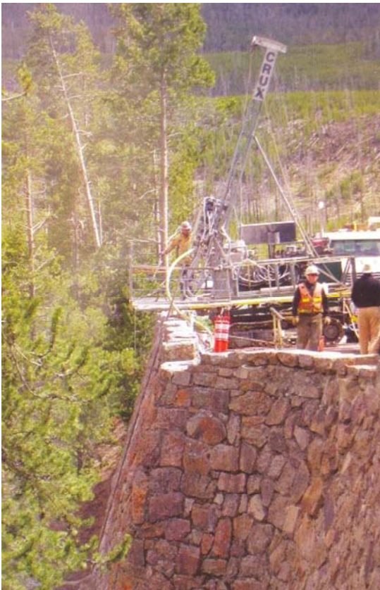
Figure 19. Micropile installation at Gibbon Falls Retaining Wall (Barrows et al., 2005).
