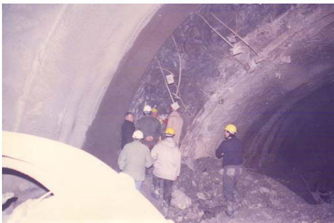
Figure 26. The maximum squeezing deformation of the Tymfristos Tunnel was as much as of 2 m.
