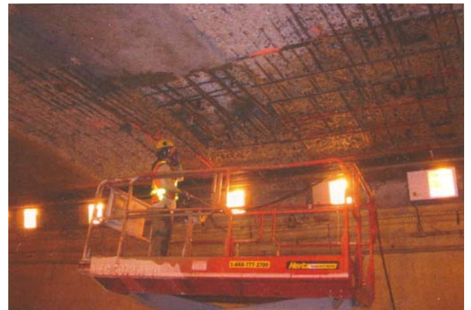
Figure 25. Crews prepare the main joint between tunnel sections for structural repair and strengthening of George Massey Tunnel.
